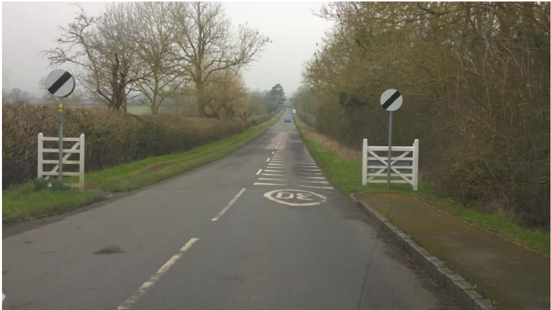
New Road – grassed over surface from Weedon
